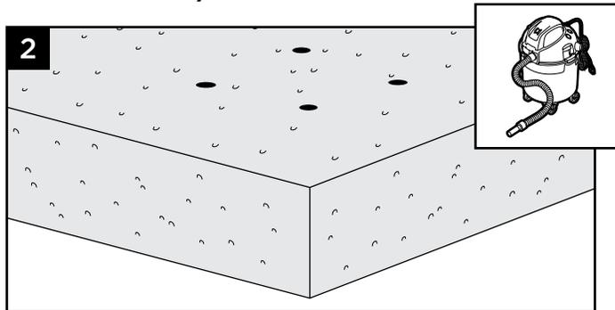
2. Clean out holes to remove all concrete dust.
