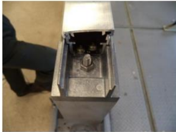
Photo No. 7 Top Rail to Post Mount Connection (Crossover Bracket)
