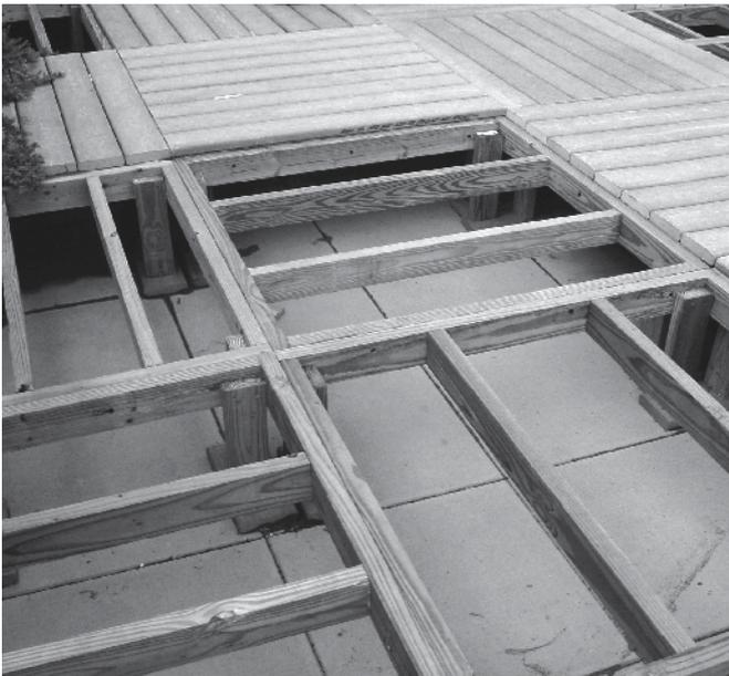
A sleeper system is a buffer between a solid surface and Trex® decking. Drainage, access, and airflow are critical. Water must be able to flow through and away from the deck. For repairs and removal of debris, joist system access is necessary. Good airflow will keep the decking dry and in good condition.
